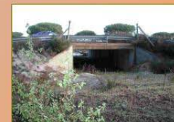
Corridors de faune Steps to fauna
