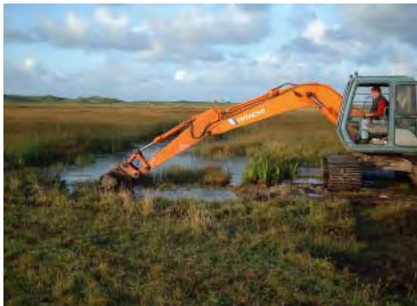
Pond excavation work in the Termoncarragh lake SPA, in Ireland.
