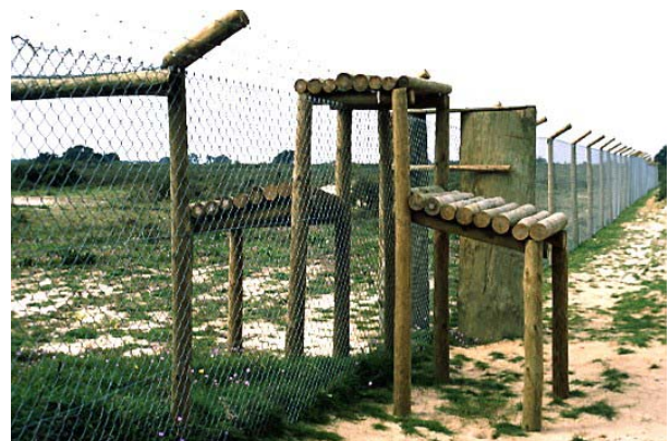
Fig. 8. Large rabbit restoration fence in the Doñana research reserve. Only lynx, but no other terrestrial predators cross the fence over this special ladder.
