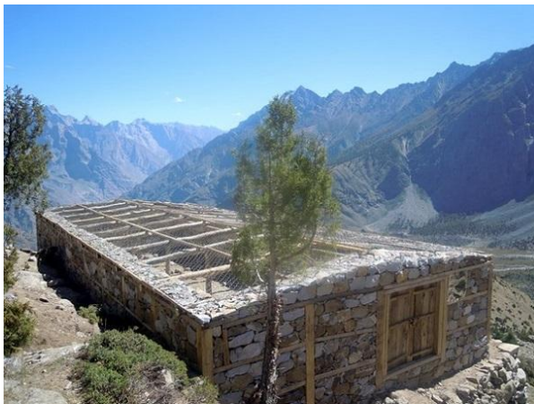
Figure 64. A predator-proof corral constructed by villagers in Baltistan, Pakistan with the aid of Project Snow Leopard and the Snow Leopard Conservancy (SLC 2017)
