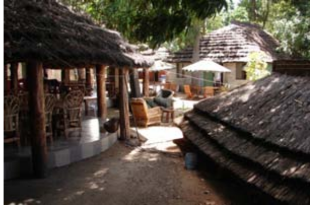
Communal area with dining room (left)
