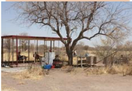
Ghanzi camp construction, before and (below) after.
